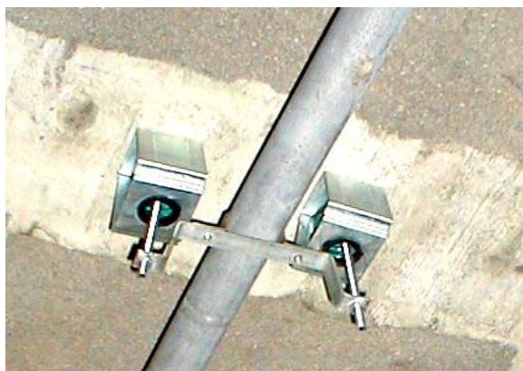
Internal spring insulator: with standard M8 (optional M10)
